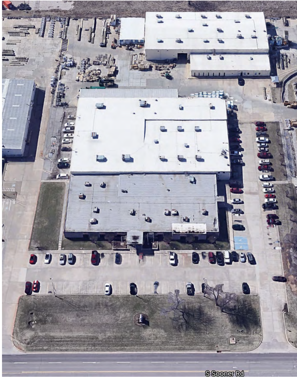
Figure 5: from the east looking west
