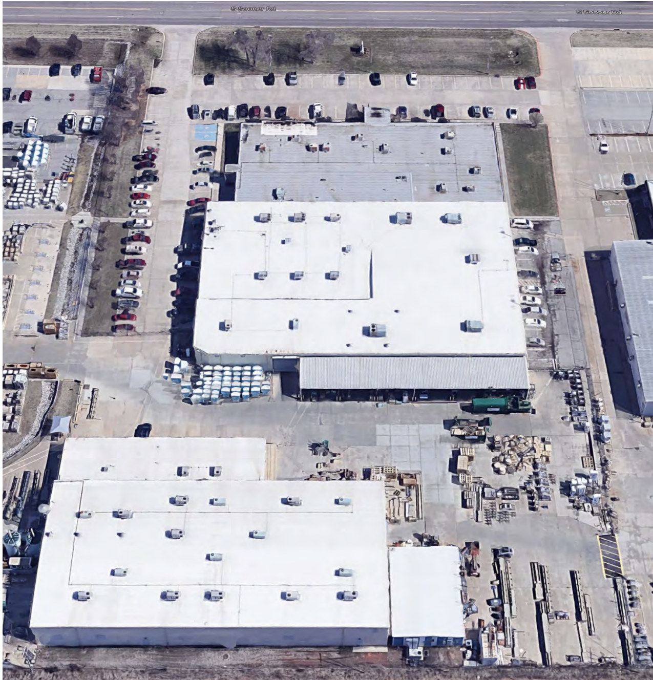
Figure 3: From the west looking east
